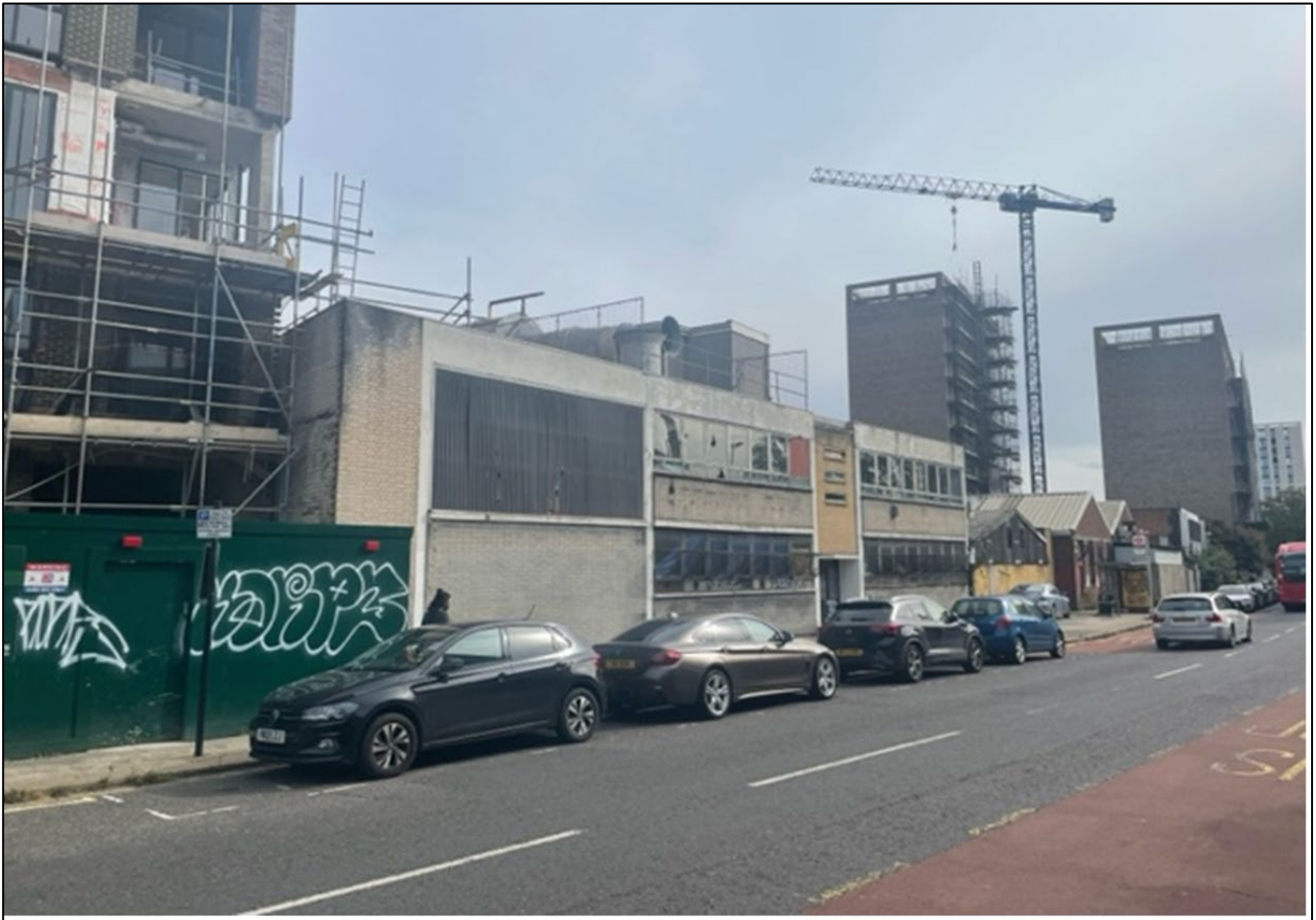
Figure 03: Existing Site Conditions for 67-81 Stirling Road (from Bollo Lane) (Block JK)
