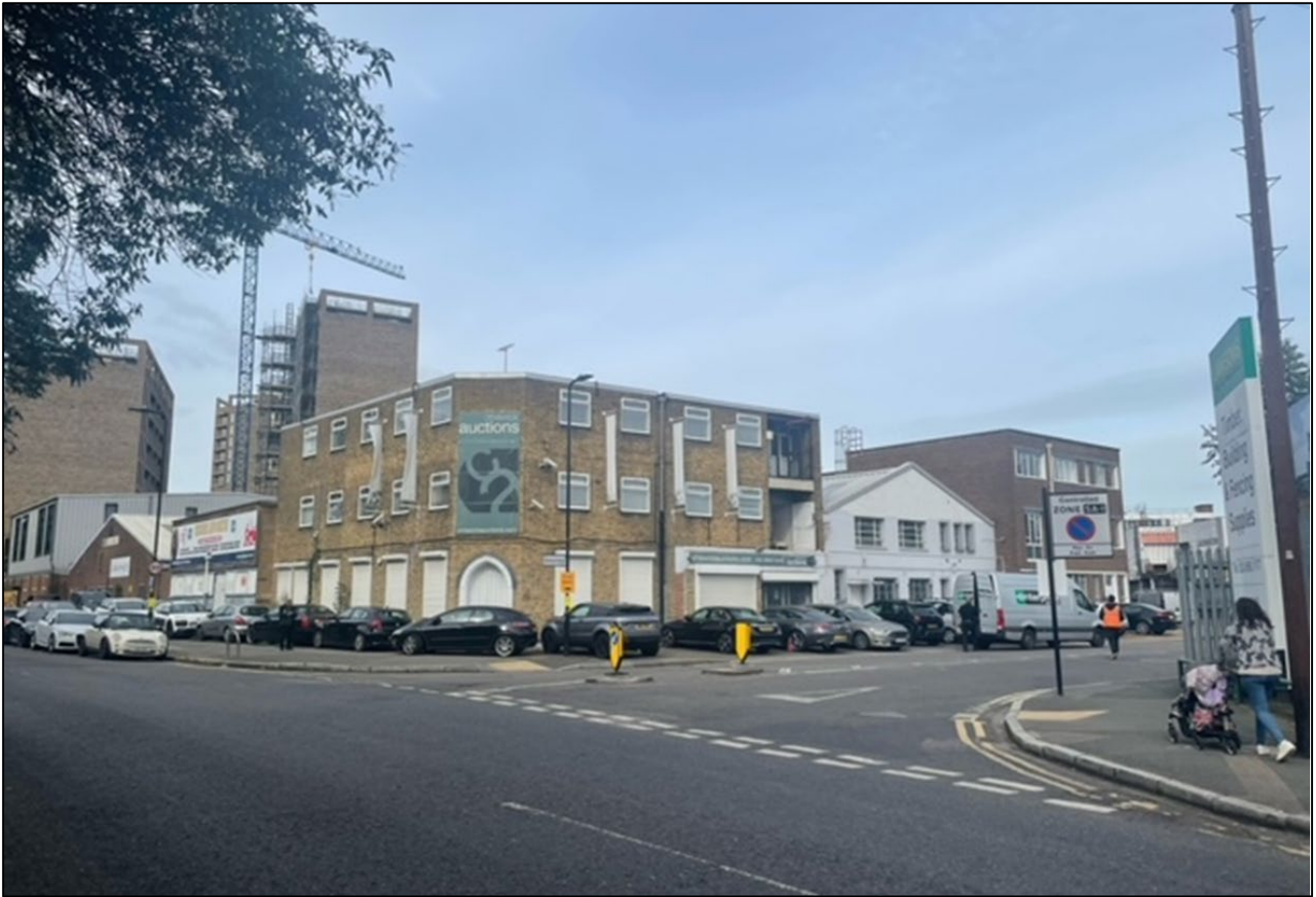
Figure 02: Existing Site Conditions for 1-9 Colville Road (Block AB)
